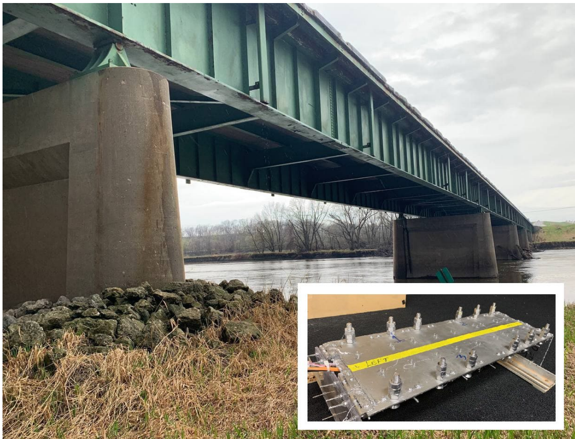
Figure 2.1 Representative bridge prototype and small-scale testbed used in the research.
